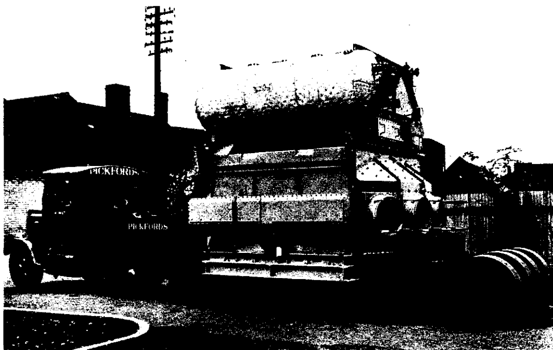
FIG. 5.—JOHN THOMPSON-LA MONT BOILER IN TRANSIT
