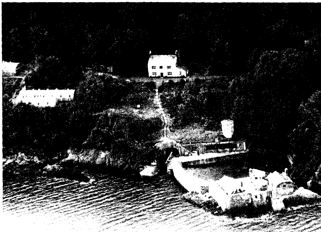
PIER CELLARS, NEAR CAWSAND—WEEKEND INITIATIVE TRAINING BASE
