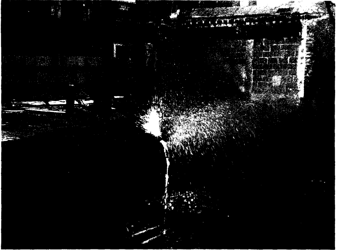
FIG. 6—CUTTING THROUGH SIX FEET OF CONCRETE
