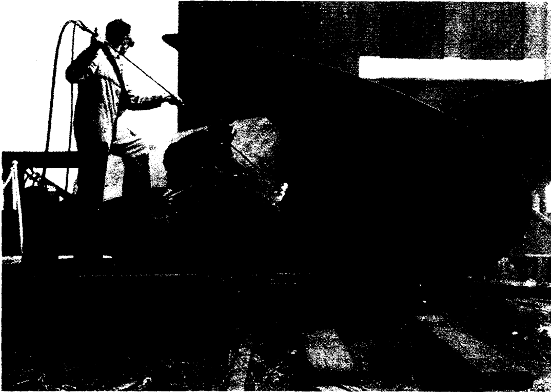
FIG. 11—POWDER LANCING A 30-TON BRONZE PROPELLER
