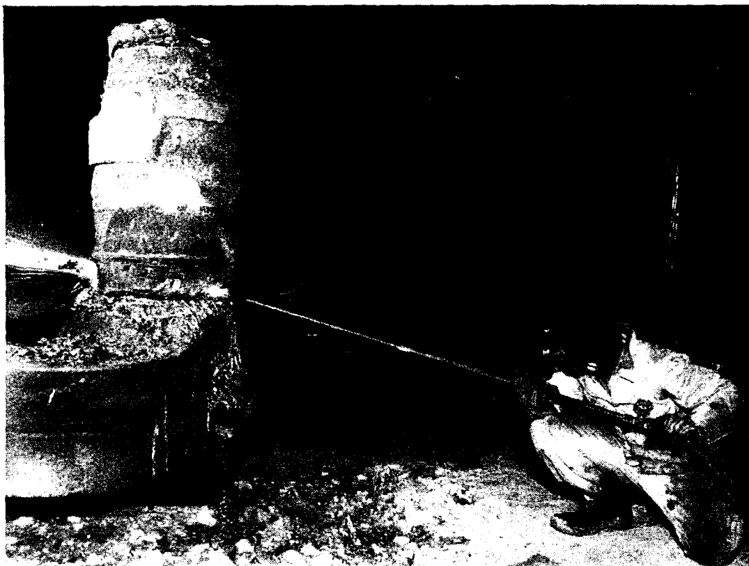
FIG. 1—REMOVAL OF HEAVY RISER FROM STEEL CASTING BY STANDARD LANCE
