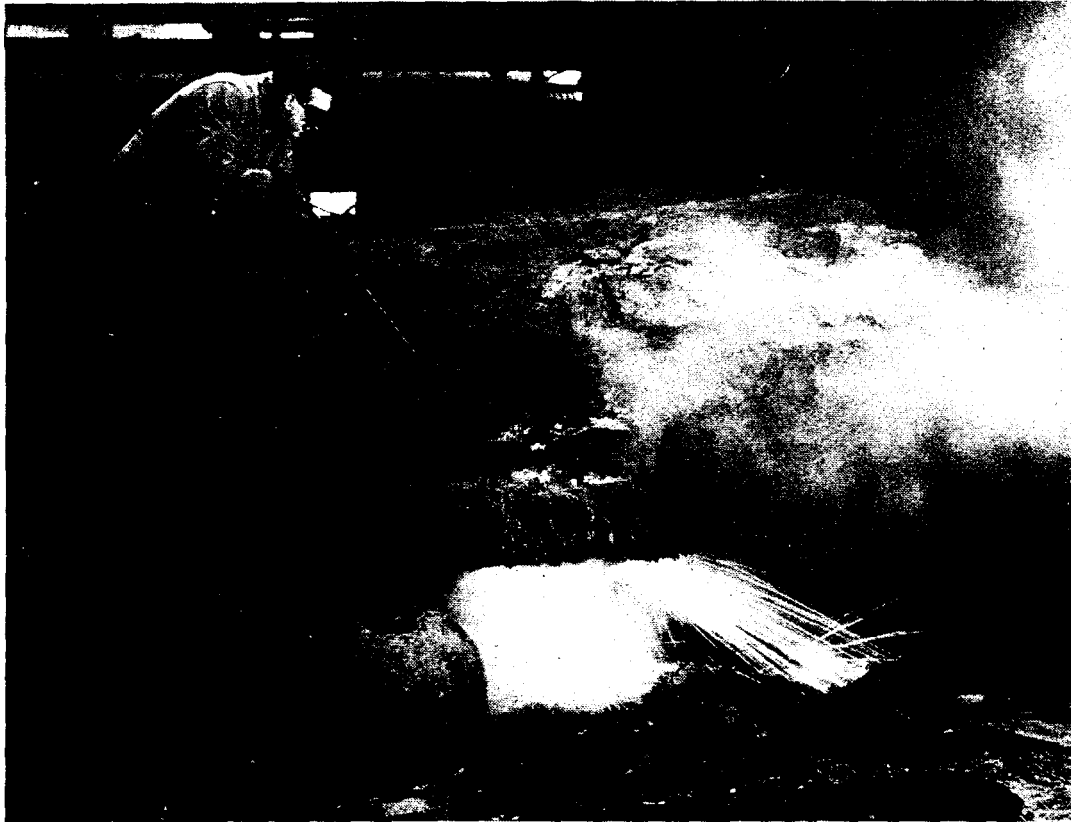
FIG. 3—THERMIC BORING A COPPER FURNACE BEAR
