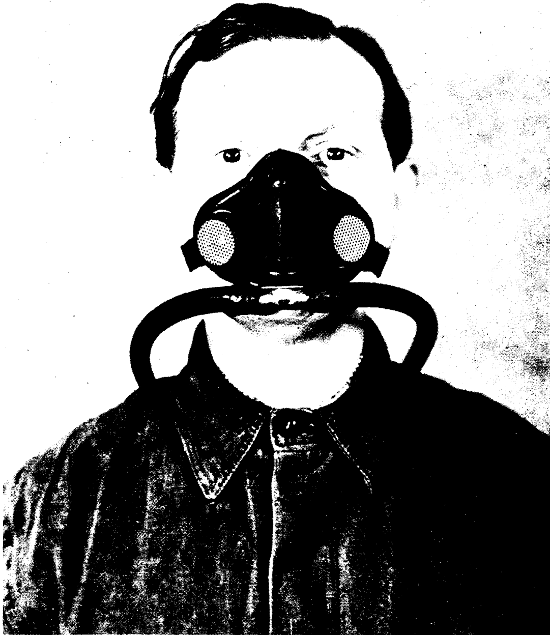
FIG. 6—SIEBE-GORMAN COMPRESSED AIR TYPE RESPIRATOR
