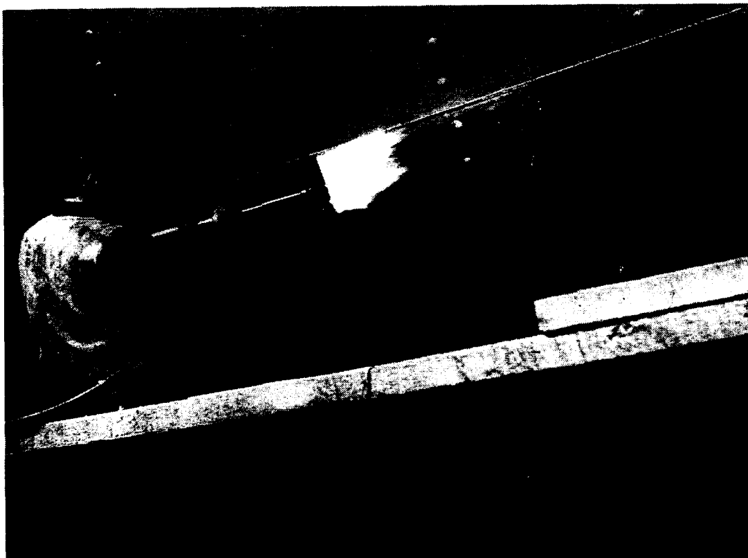
FIG. 3—FLAME CLEANING THE SIDE OF A CARGO VESSEL AT MESSRS. JOHN BROWN LTD., OF CLYDEBANK
