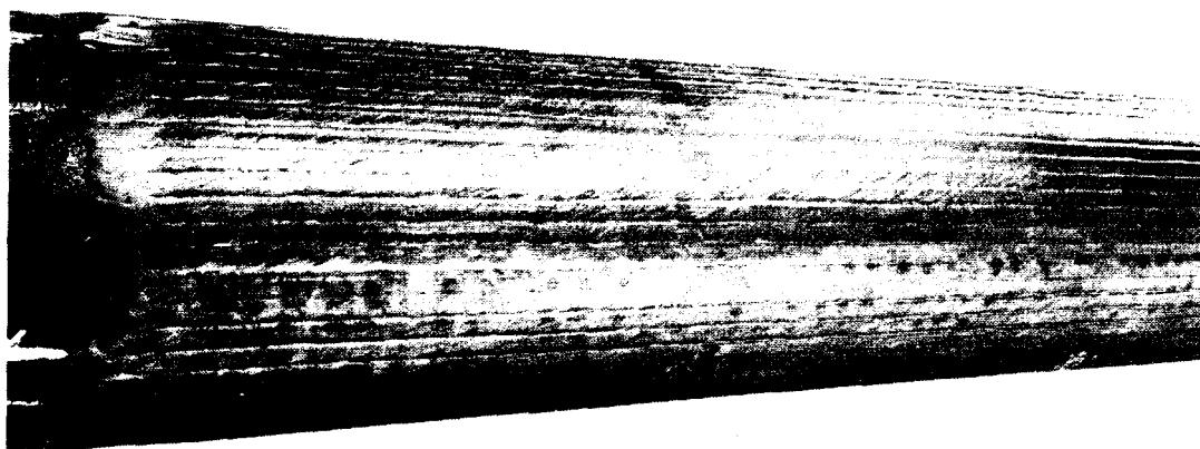
FIG. 11—WELDING COMPLETED. THE REINFORCEMENT IS TWO LAYERS HIGH
