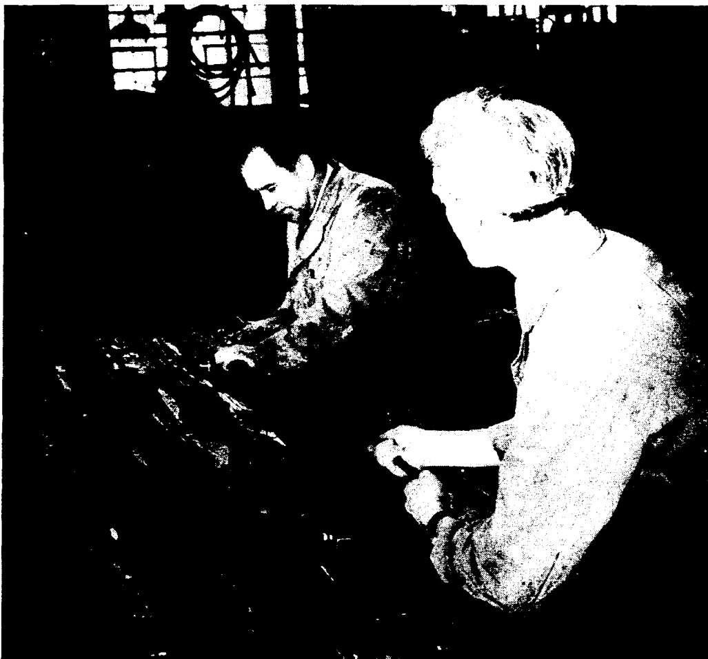
FIG. 2—THE ROLLERS BEING PULLED ALONG A TUBE. NOTE THE CLAMPS FITTED TO PREVENT THE SHEET PULLING AWAY FROM A COMPLETED TUBE
