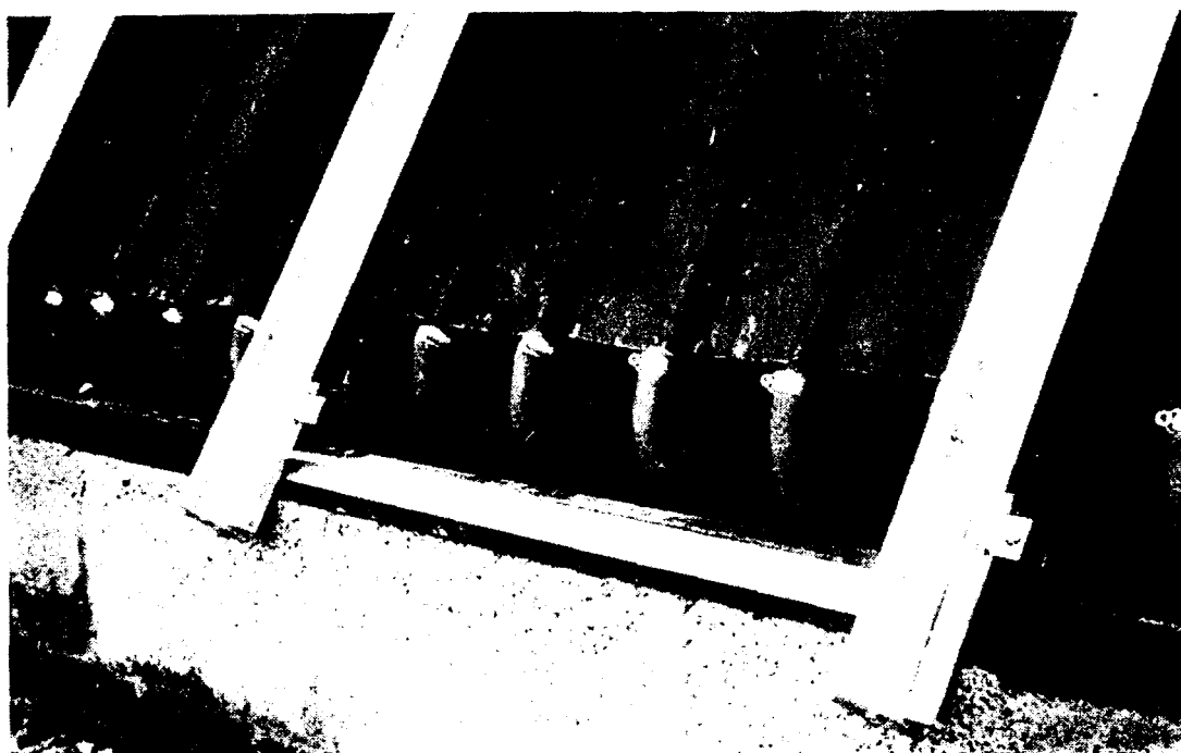
FIG. 5—CLOSE-UP OF THE ENDS OF TWO GLAZING BARS WITH A DRAUGHT EXCLUDER STRIP BETWEEN THEM
