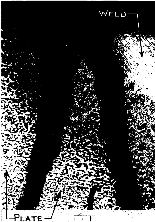
FIG. 14—ORIGIN OF FISSURE SHOWN IN FIG. 13
