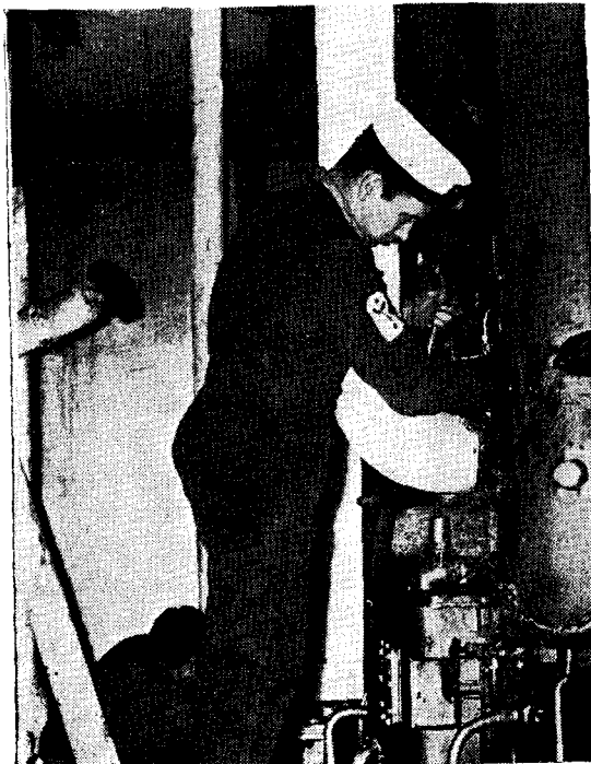
FIG. 3—RATING AT WORK IN Y.102 BOILER ROOM
