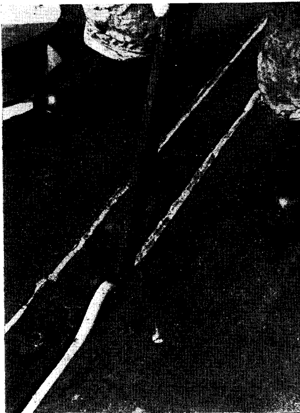
FIG. 2—CAULKING REMAINING GAP BETWEEN RETAINING BAR AND FLIGHT DECK
