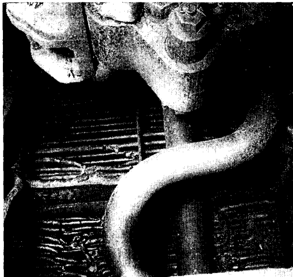
FIG. 4—CONDENSER SHOWING SOME OF THE DAMAGED TUBES
