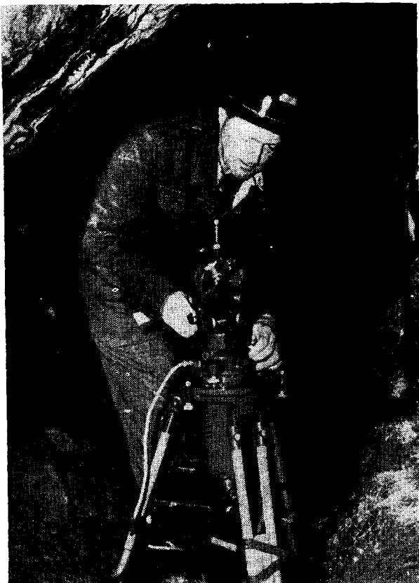
FIG. 3—PIM BEING SET UP FOR USE IN TUNNEL ALIGNMENT
