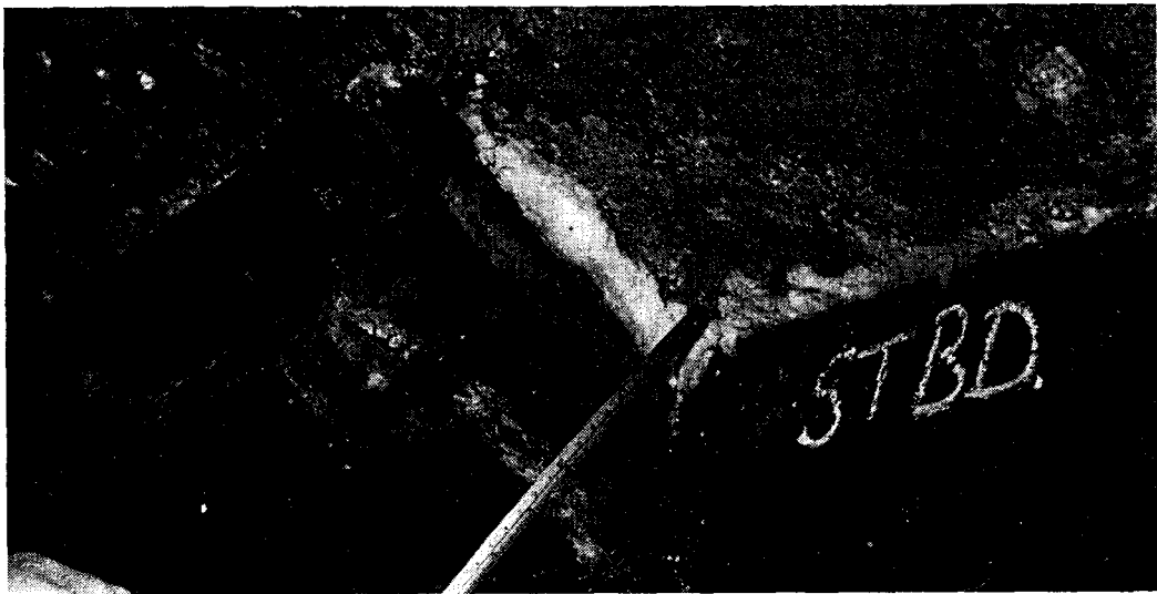
FIG. 8—SECTION OF GARBOARD STRAKE HAO deposits are forcing it away from the keel-plate and pulling the securing bolts through.
