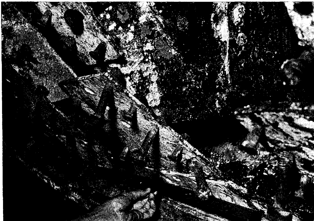
FIG. 6—SECTION OF KEEL ANGLE Distortion due to build-up of HAO between aluminium and hull planking.
