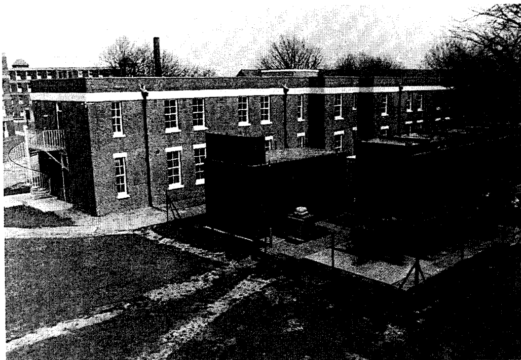
FIG. 3—AERIAL VIEW OF THE SEWAGE TREATMENT PLANT TRIALS FACILITY AT H.M.S. 'SULTAN'. FROM LEFT TO RIGHT: 'SULTAN' ACCOMMODATION BLOCK AUXILIARY MACHINERY AND COLLECTION PLANT ACOUSTIC ENCLOSURE AIR OUTLET WITH FILTRATION EQUIPMENT END OF INSTRUMENTATION CABIN ISO CONTAINER ON ITS ROLLING PLATFORM
