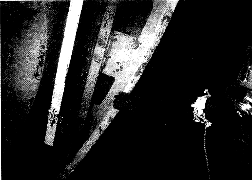
FIG. 6—LOWER END OF AFTER SHORE. THE SHORE WAS PREVENTED FROM MOVING OUT BY THE LIP OF THE BOW DOOR OPENING
