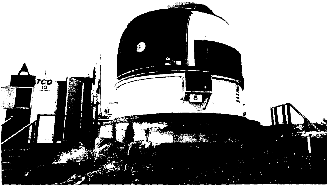
FIG. 3—THE CINE-SEXTANT OPTICAL TRACKING SYSTEM ON WINCHELSEA ISLAND
