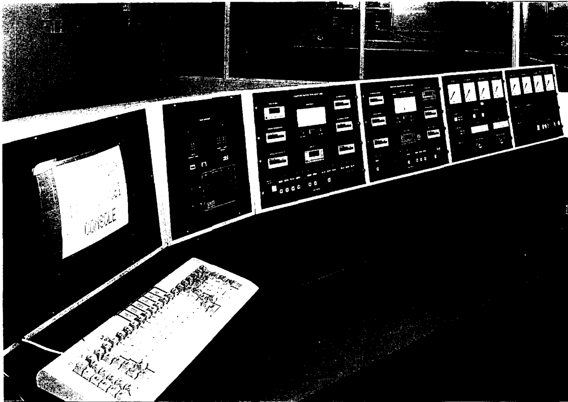
FIG. 8—THE CONTROL CONSOLE
