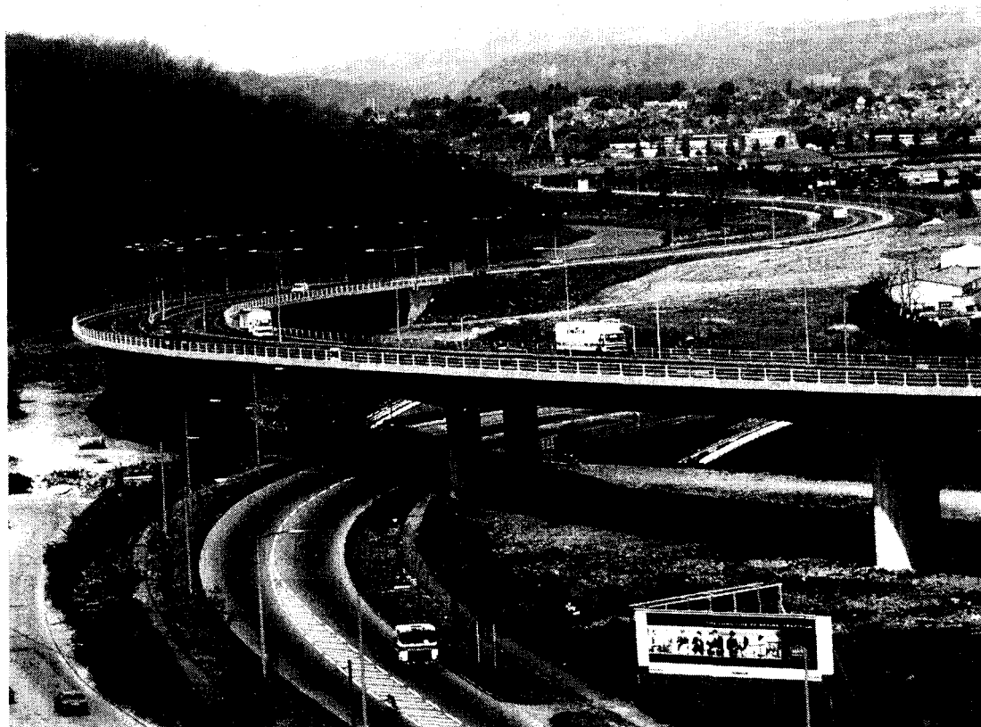
FIG. 44—SEGMENTAL PRE-STRESSED CONCRETE VIADUCT
