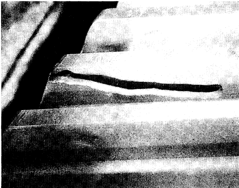
FIG.4 – NDE WHILST REMOVING A CRACK
