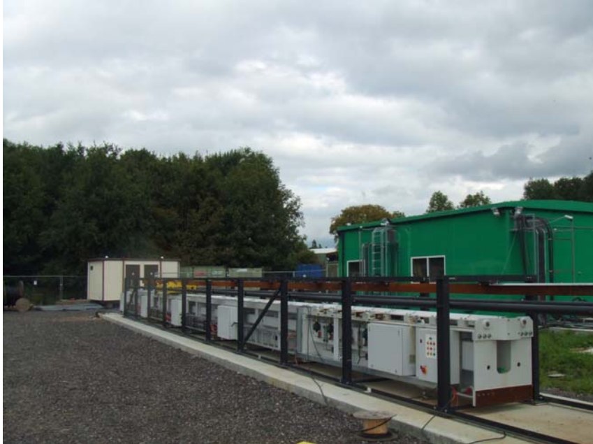
FIG.6 – EMKIT TECHNOLOGY DEMONSTRATOR SHOWING LAUNCH TRACK IN FOREGROUND
