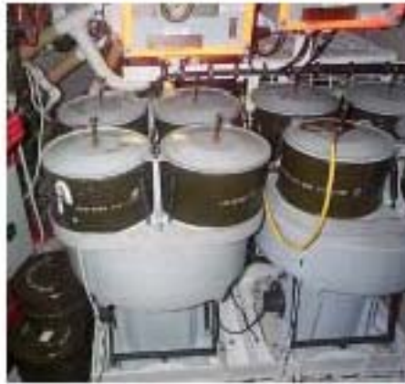
FIG.1 - CDAUS IN THE FWD ESCAPE COMPARTMENT OF A SSN. EACH CDAU HOLDS 4 CANISTERS
