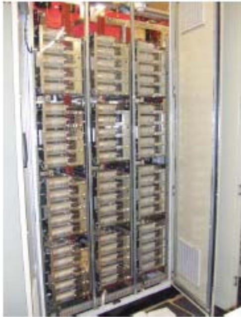
FIG.5 - CAPACITOR MODULES OF SINEWAVE FILTER
