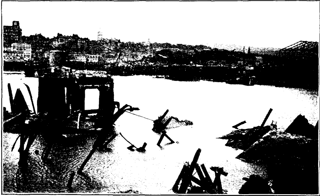
FIG. 4.—BOULOGNE. WRECKED HARBOUR INSTALLATIONS, DEMOLISHED E-BOAT PENS ARE IN THE FOREGROUND
