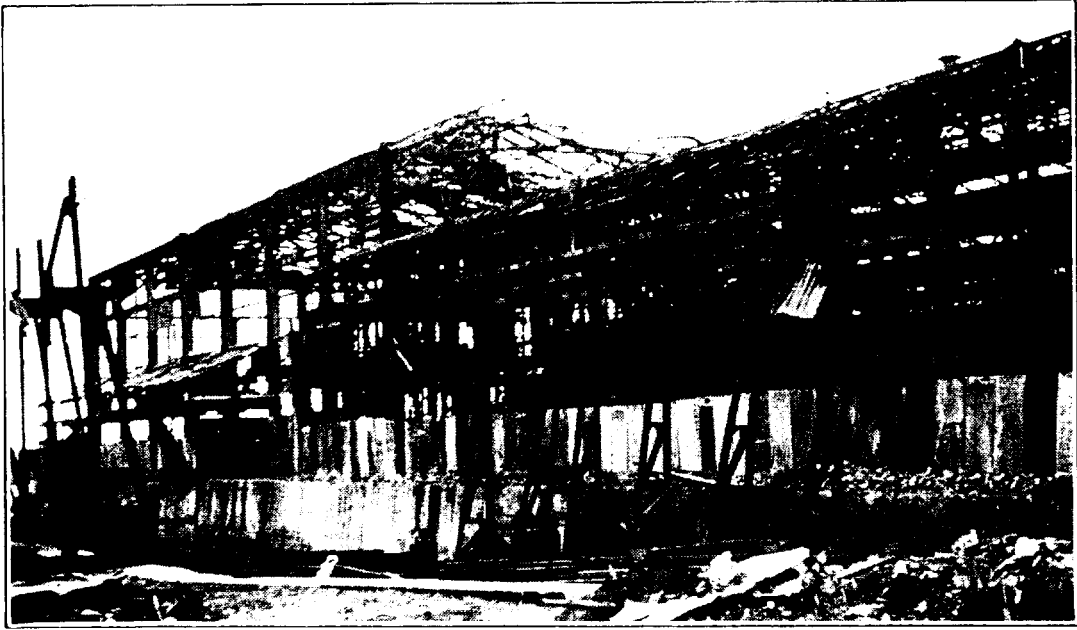
FIG. 3.—BOULOGNE. SHIP REPAIR SHOPS AND SLIPWAY DAMAGED BY R.A.F. RAIDS
