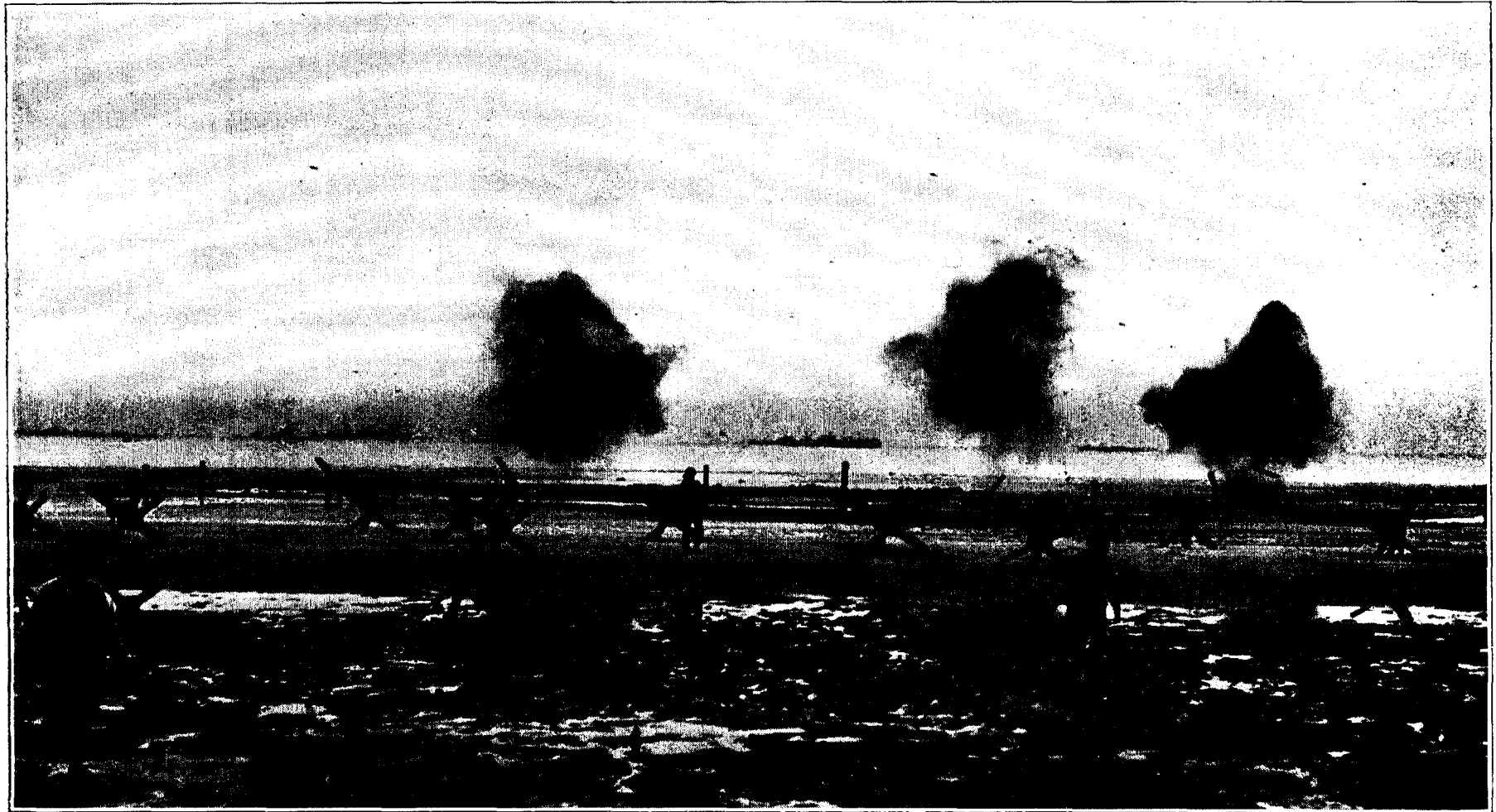
FIG. 1.—DEMOLITION OF BEACH OBSTACLES SHORTLY AFTER H-HOUR
