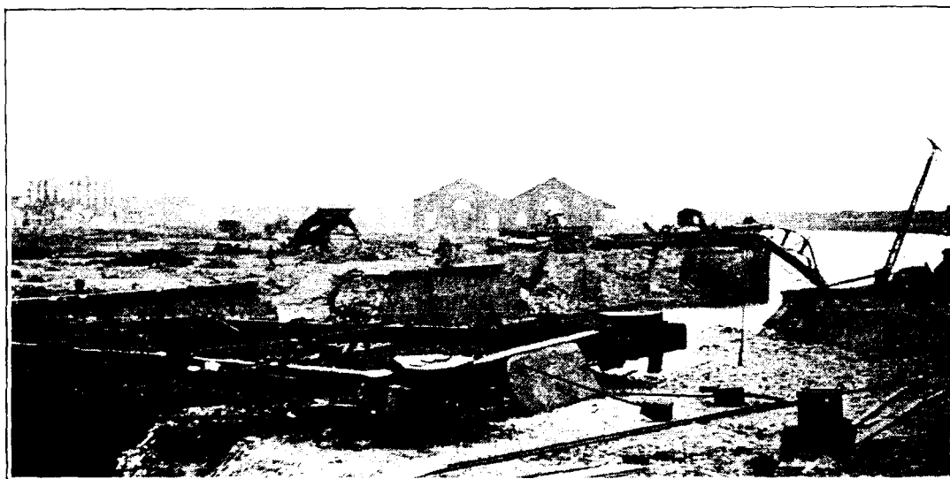
FIG. 5.—CALAIS. DEMOLISHED DOCK AREA
