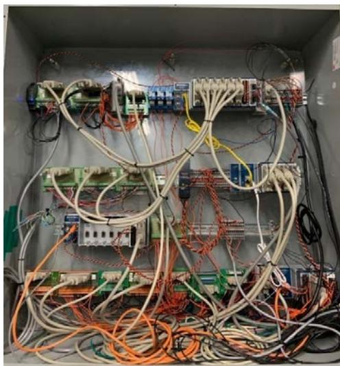
Figure 13: Cabinet housing the four NI cDAQ chassis providing overarching control of the different power supplies, Mosebach loads, MV6000, and M-G set.
