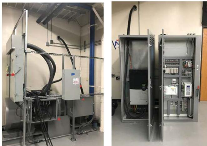
Figure 3: Photographs showing the M-G set (left) and internals of the control and VFD cabinets (right).
