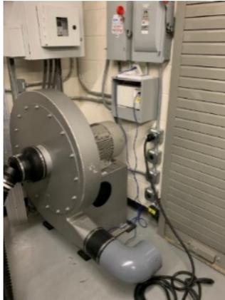
Figure 8: Photograph of the 15 HP blow, variable frequency drive, and braking resistor used to apply forced air cooling to the 4160 VAC transformer and 4160 VAC/ 6 kVDC rectifier.
