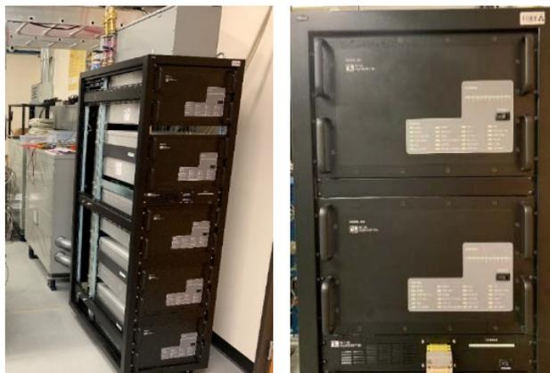
Figure 10. Photograph showing the two – 40 kW power supplies used to convert 480 VAC to 12 kVDC (upper two supplies) and the three – 50 kW power supplies used to convert 480 VAC to 1.2 kVDC (lower three supplies).
