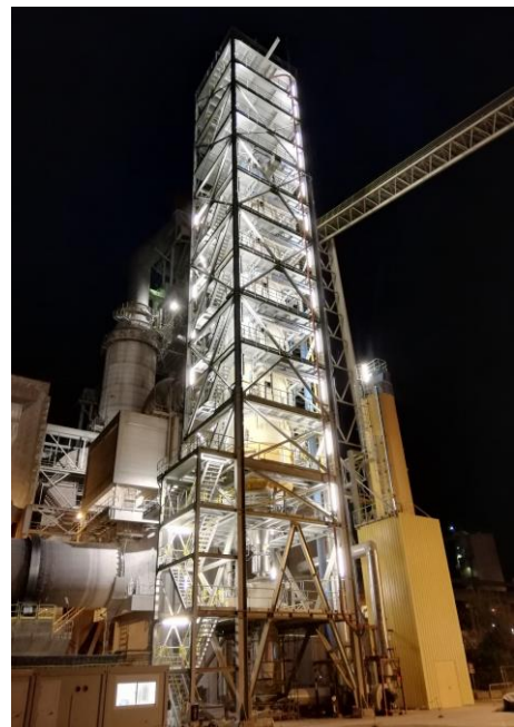
Figure 2: The LEILAC1 Pilot Plant for low emissions Lime
