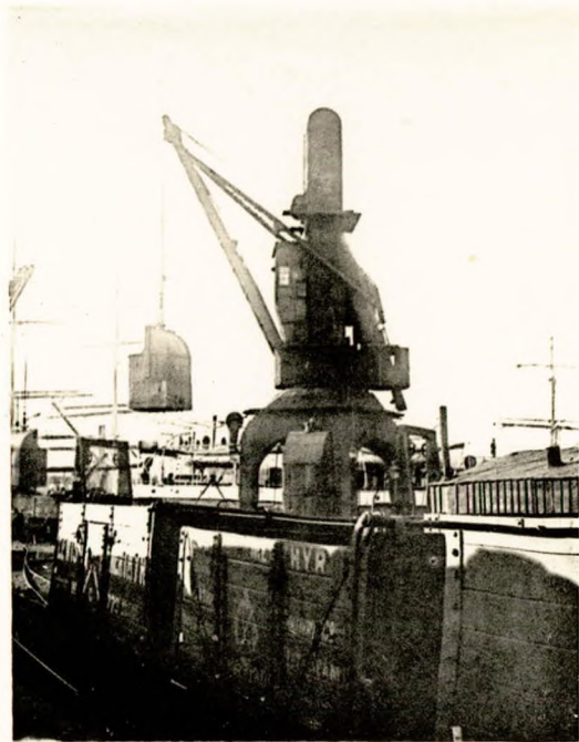
Fig. 36. NEW HYDRAULIC COALING CRANES, BUTE DOCKS, CARDIFF.
