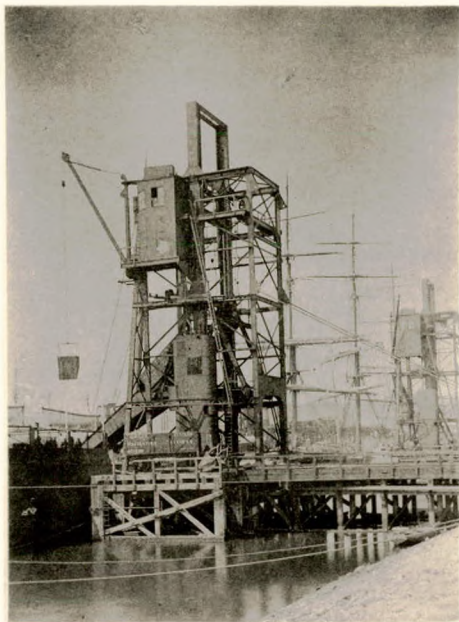
Fig. 31. LOW LEVEL, HYDRAULIC COAL TIPS, BARRY DOCK.
