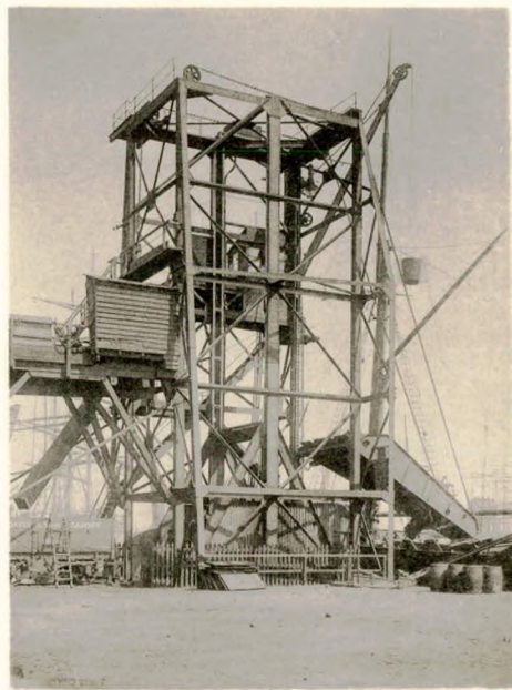
Fig. 30. HIGH LEVEL, HYDRAULIC COAL TIPS, BARRY DOCK.
