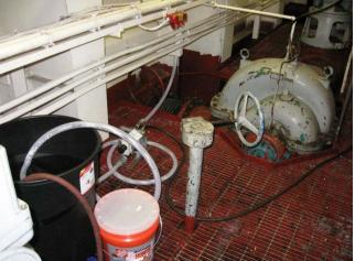
Photo 7 - Inline dosing setup
