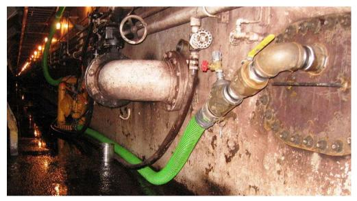
Photo 21 - Chemical injection manifold tee fitting shown, transfer pump in background
