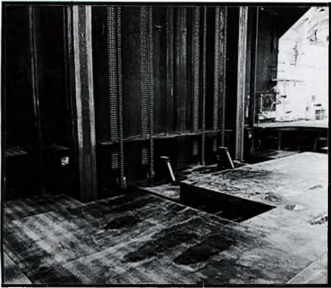
Fig 6: Aft aircraft lift recess hangar deck
