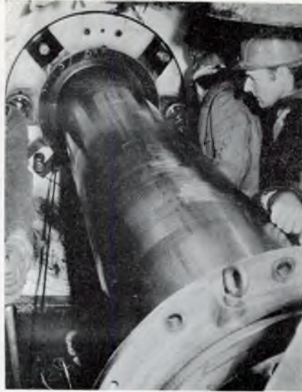
FIG. 8 (Left)—Commencement of the withdrawal operation FIG. 9 (Right)—Withdrawal of the bearing: the inboard seal has been removed along the shaft. The bearing has been jacked clear of its seating and is now being winched along the shaft.
