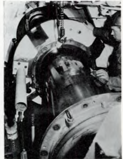
FIG. 12—Replacement of bearing
