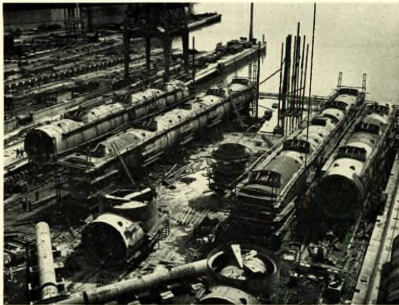
FIG. 20—Construction of Staflo semi-submersible
