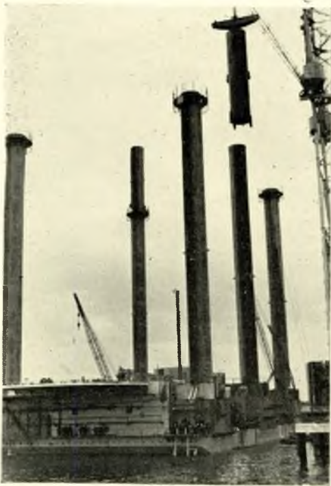
FIG. 11—Self-elevating outfit—Placement of leg section
