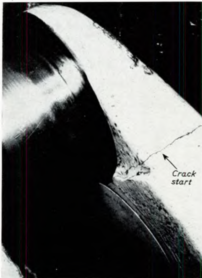
FIG. 19—Fracture initiated at the edge of the crankweb of a small, cast steel crank throw (semi-built)
