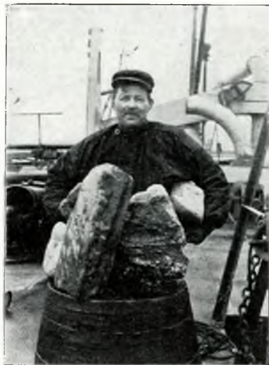
FIG. 41—Stones sucked into suction pump of suction dredger
