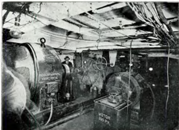
FIG. 42—Electric drive of suction pumps in suction dredger (1921)
