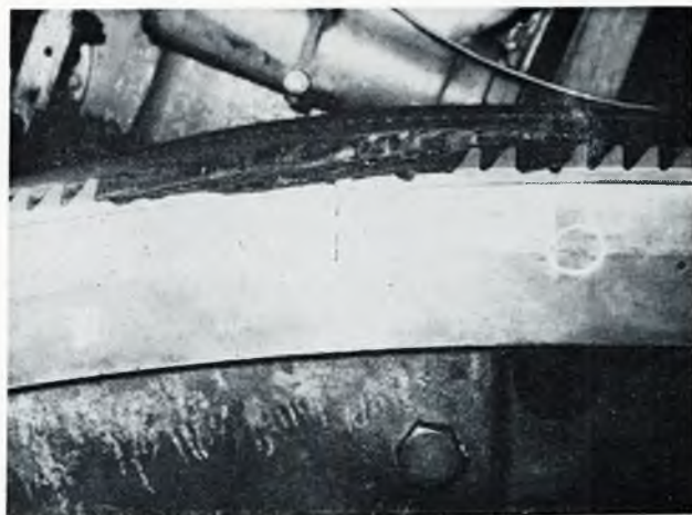
a. Cracked rim of bull-gear wheel.
