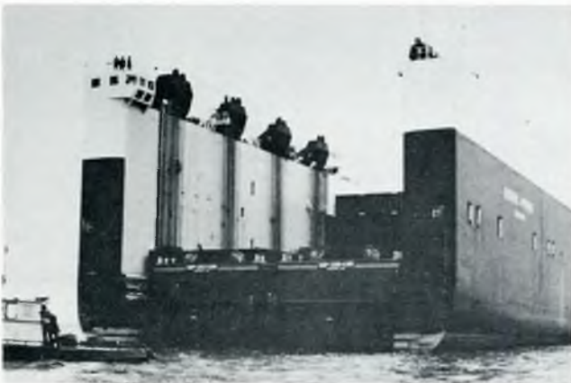
FIG 2 View of cantilevers with barges lifting platform and hoisting machinery
