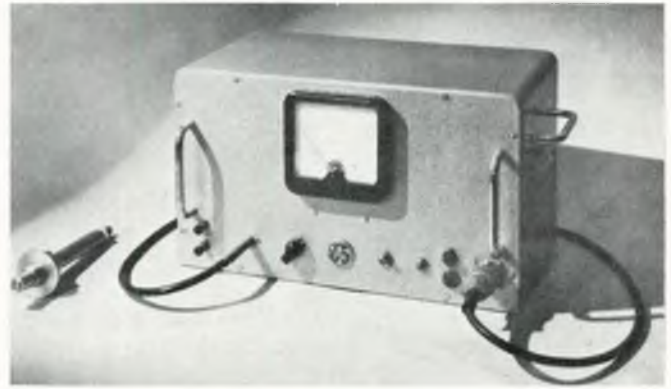
FIG. 4—Capacitance clearance monitor
