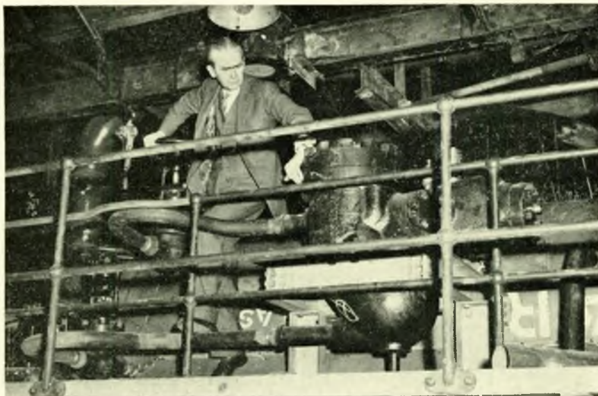
FIG. 20—An example to illustrate the large size of conventional steam fittings
