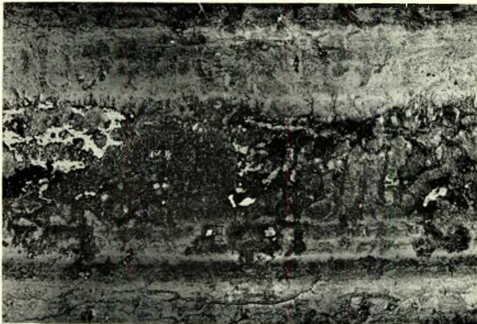
FIG. 29—Furnace cracking due to oil contamination
