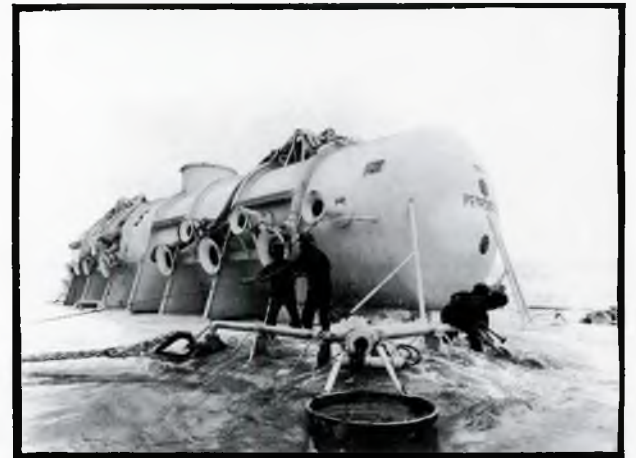
Fig 15: Petrobras Garoupa subsea production system
