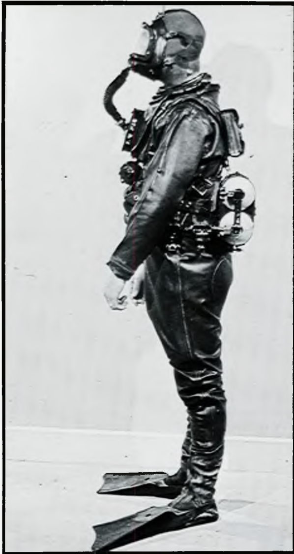
Fig 13: Royal Navy clearance diving breathing apparatus (1960)
