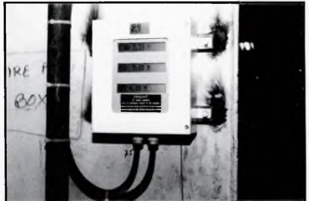
Plate 1: Reading from an automatic draught gauge More information is now displayed in the same space.
