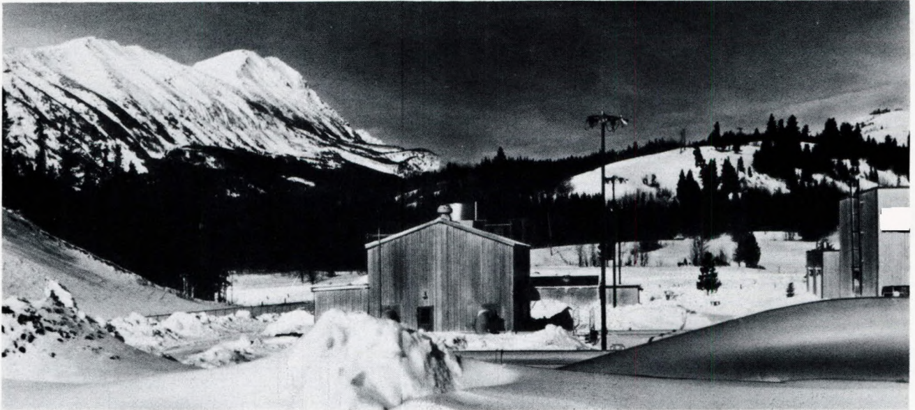
FIG. 7 A typical Avon gas pumping station on a natural gas pipeline in Alberta, Canada
