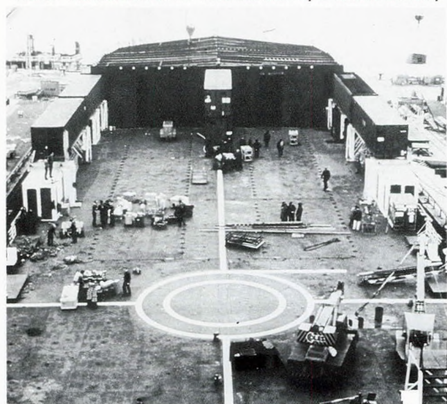
FIG. 6 Conversion of MV Atlantic Conveyor to aircraft ferry
