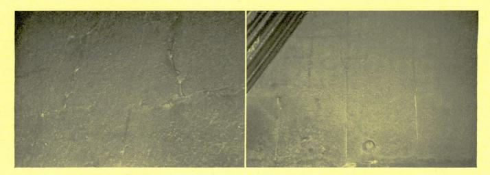
FIG. 20 Front walls above burners in controlled superheat boilers showing very little damage after two years' service
