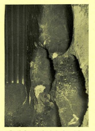
FIG. 25—Burner quarl section in a D-type boiler (four years' service)
