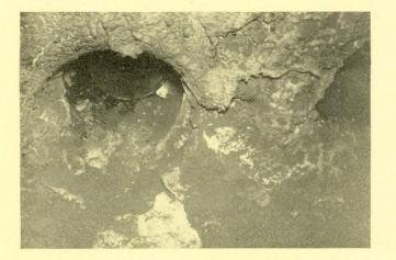
FIG. 22—Burner quarls in very bad condition after three years' service due to poor maintenance
