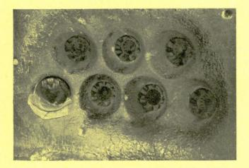
FIG. 19—Burner arrangement in a controlled superheat boiler showing dish shape including quarl tubes
