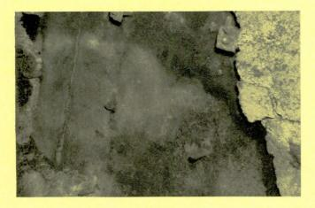
FIG. 18—Back wall of single-pass header type boiler stripped for replacement of rammed plastic lining (four years' service). Note burned-off anchor bolts
