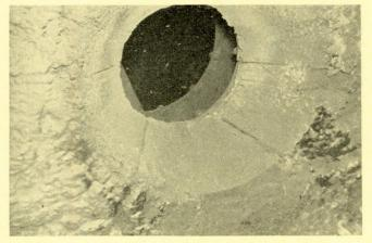
FIG. 24—Burner quarl in good condition after four years' service
