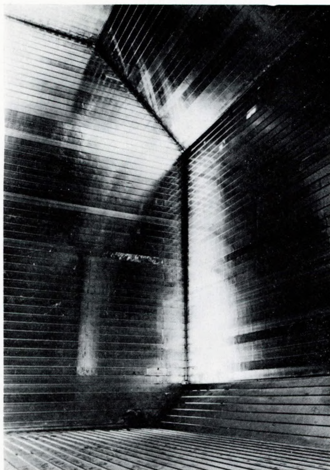
FIG. 4—Internal view of Invar membrane tank on Polar Alaska
