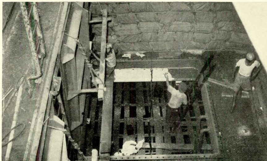
FIG. 12—Wax coating of hatch coaming in progress
