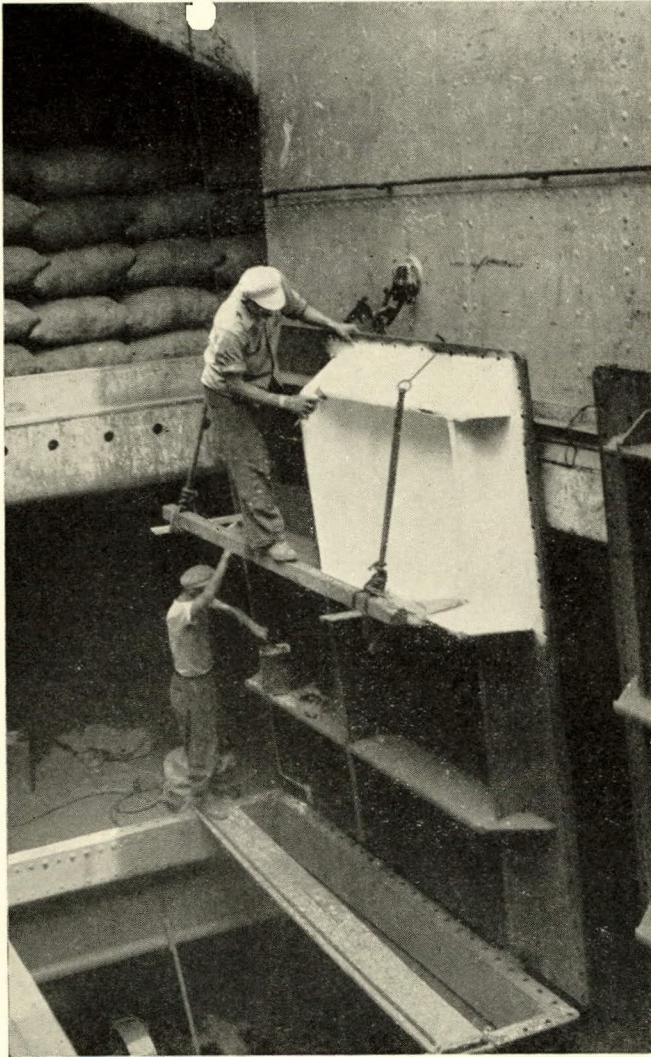
FIG. 13—Wax coating of hatch cover in progress
