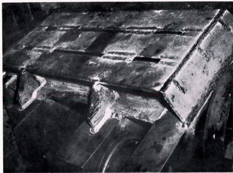
FIG. 7—Prefabricated girders fitted across crankwebs
