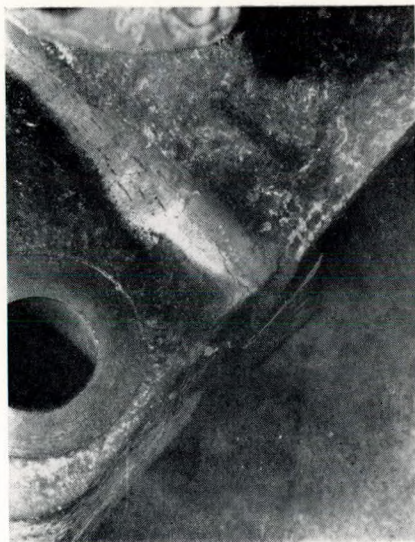
FIG. 28—Top half of h.p. cylinder: view of defect "D"
