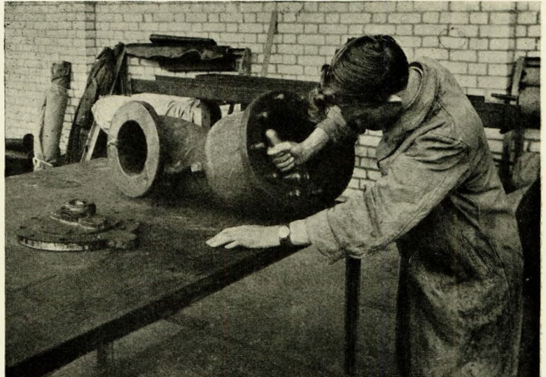
FIG. 13—Lining the interior of a seacock casing with rubber With acknowledgements to "Shipbuilding and Shipping Record"
