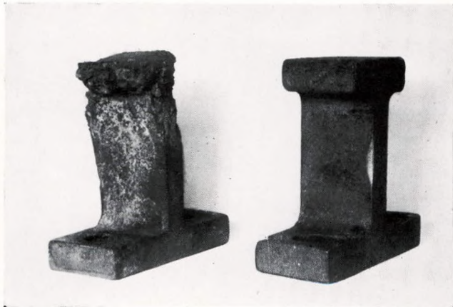
FIG. 9—Wastage of cast-iron brick key
