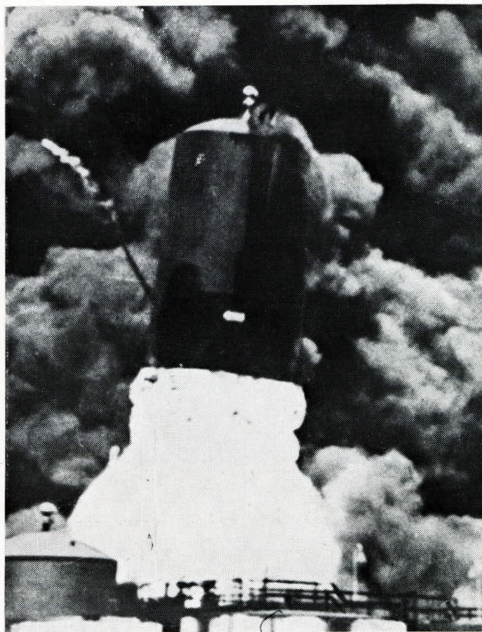
FIG. 12— Exploding asphalt tank
