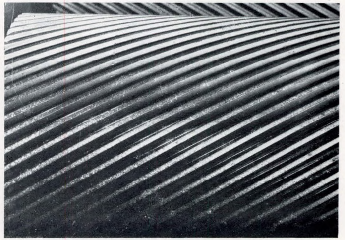
FIG. 11.—Unprotected starboard engine surfaces rusty
