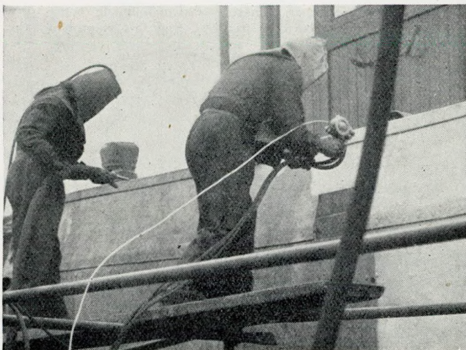
FIG. 1.—Sand blasting and zinc spraying a steel hull
